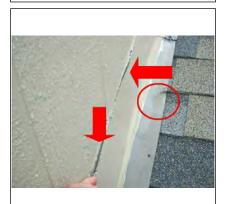
Gaps at chimney flashing, nail heads not sealed.
