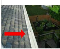
Rear leaf guard should be installed under shingles, nail heads will cause leaks.
