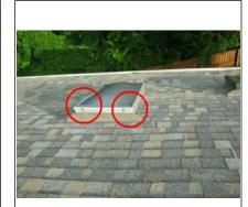
Rusted fasteners on skylights, galvanized or stainless required
