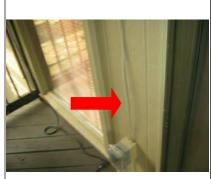
Cable for upper rear outlet must be in a conduit
