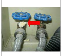
Clean and monitor washer corroded connections.
