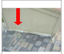
Poor flashing detail at chimney chase, open gaps at top.
