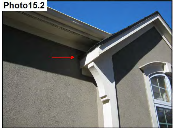
Seal open gaps.
