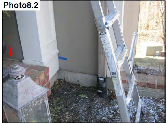
EIFS in contact with brick
