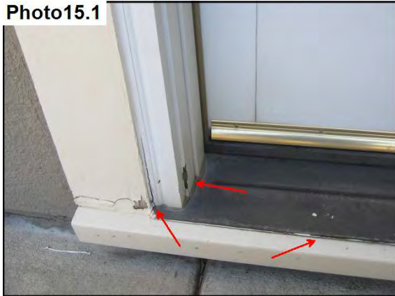
Seal all thresholds
