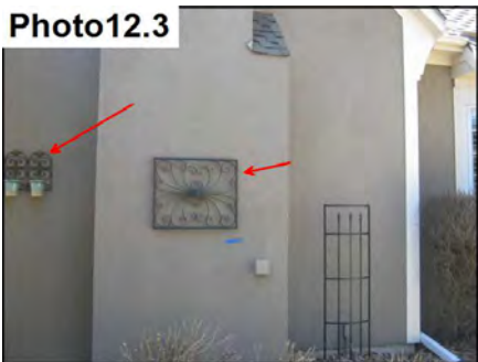
Improper attachment
