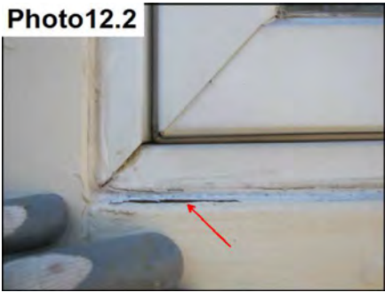
Inadequate sealant
