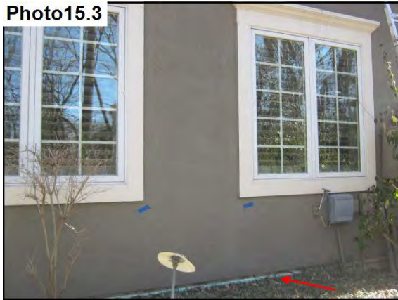
Good clearance to grade
