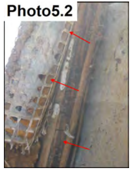
Plywood, yellow insulation, white mesh.
