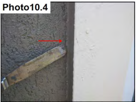
Missing sealant.
