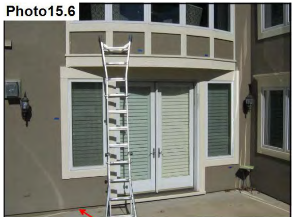
Good clearance to rear patio
