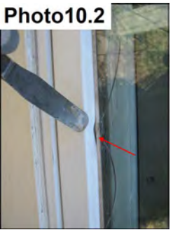
Cracked window bent metal cladding lower window
